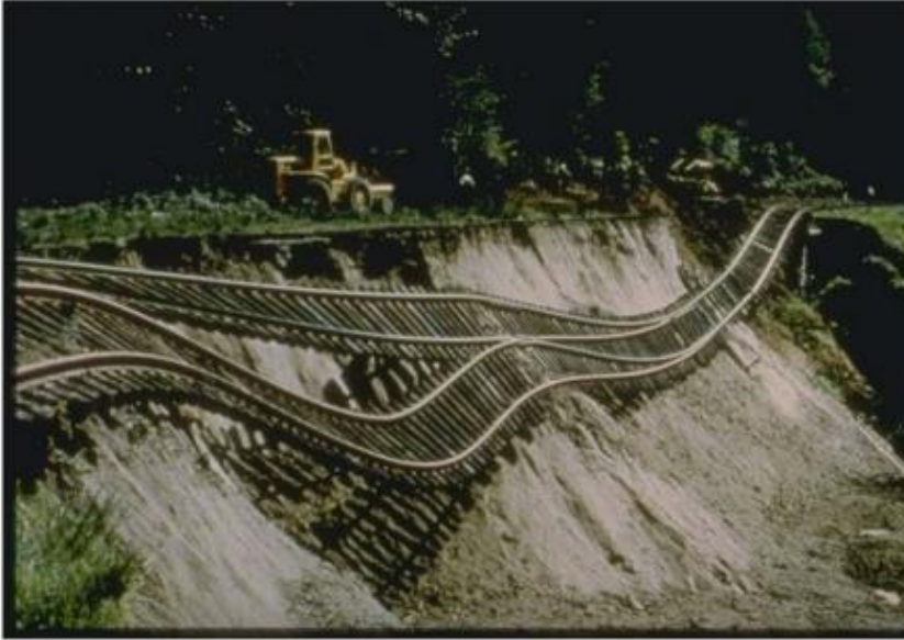
Figure 3: During the 1965 Puget Sound Earthquake, a large portion of the railroad lines north of the old brewhouse were significantly damaged in an earthquake induced landslide.
