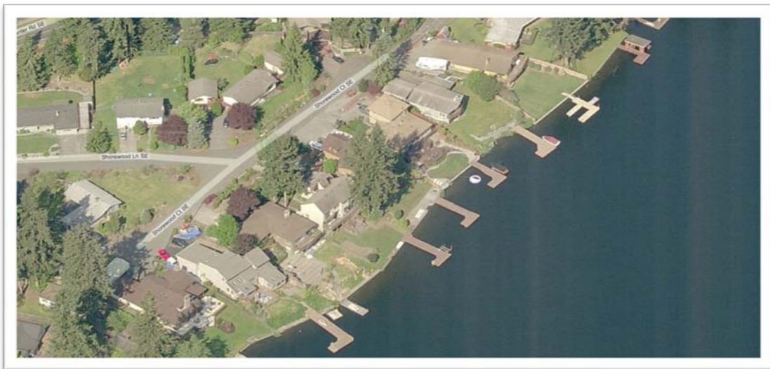
Docks and bulkheads lead to cumulative impacts on lake health. Long Lake, Lacey
